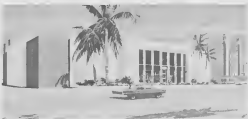
The Refining Controlhouse now being expanded contains six process computers to control the operations of practically all refinery units. It's scheduled for completion this month.
